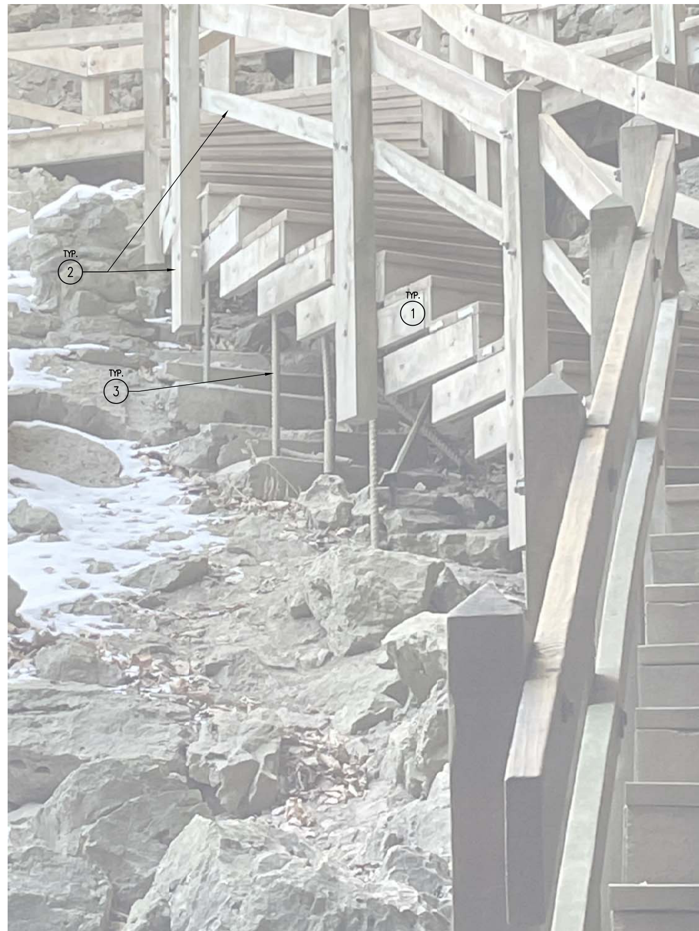
01 PHOTO – CLOSE-UP MIDDLE DANCE HALL STAIR SCALE: NTS
